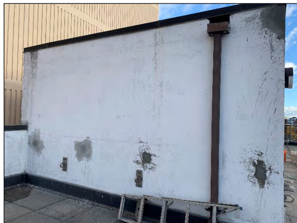
Concrete repair material placed on removed form ties at staircase enclosures.
