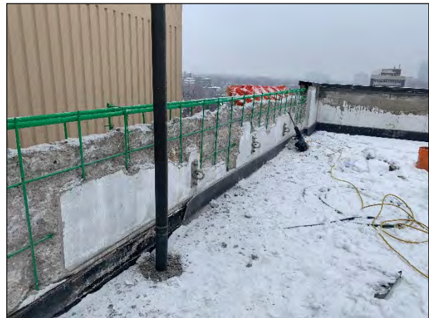
Repainting localized concrete repairs on east end of north parapet wall and north end of east parapet wall to match existing.
