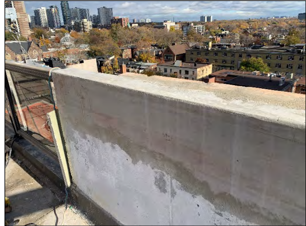
Epoxy coating application at east end of north parapet wall.
