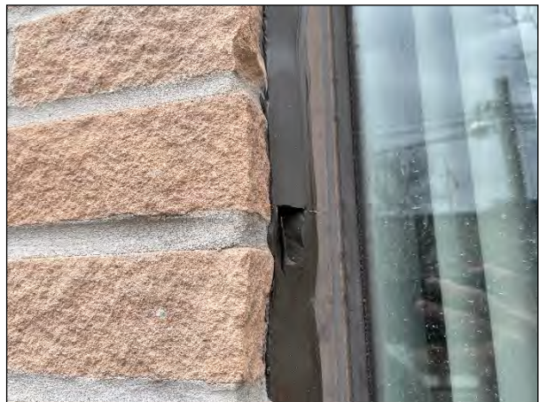
Test cuts in new sealants were conducted, and removed sealants were repaired.
