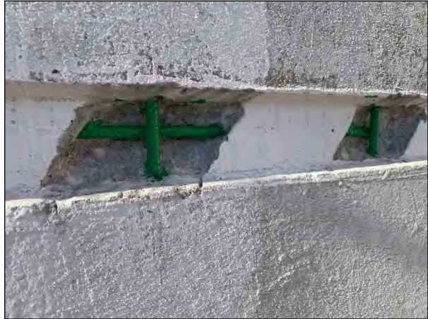
Removal of concrete wall form ties on staircase enclosures.
