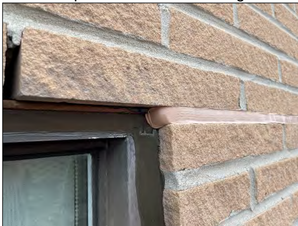
Installation of new sealants at window perimeters and soft joints along southern drop on east side of building.
