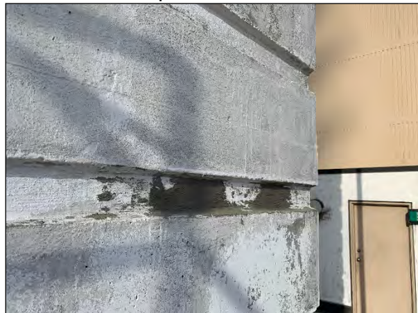
Concrete repair material placed on removed form ties at staircase enclosures.
