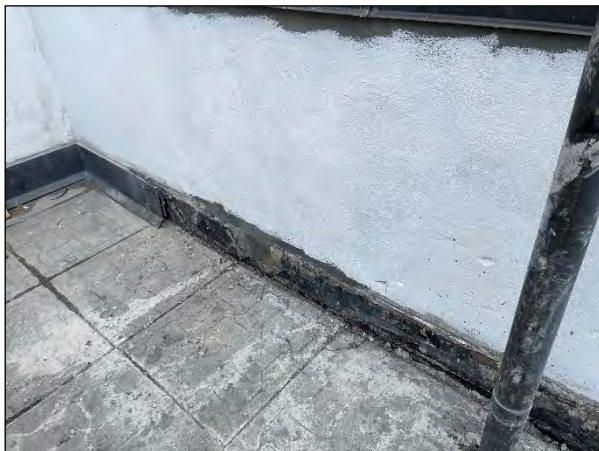
Concrete repair material placed at north end of east parapet wall.
