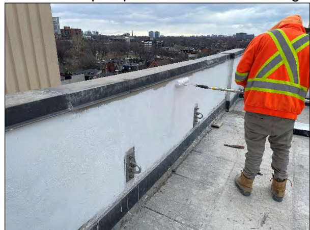
Repainting localized concrete repairs on east end of north parapet wall and north end of east parapet wall to match existing.
