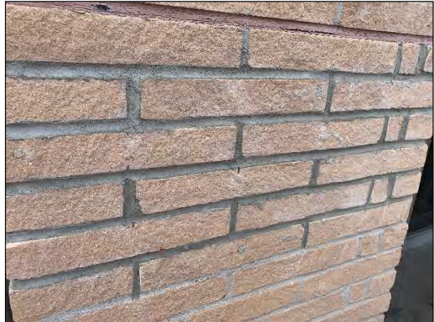
Test cuts in new sealants were conducted, and removed sealants were repaired.
