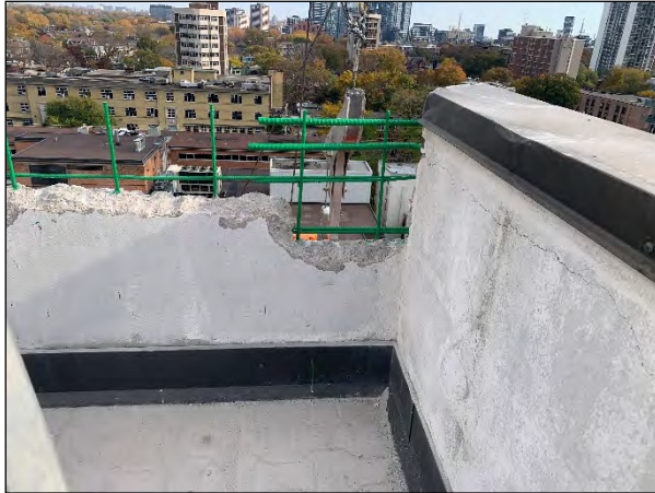
Concrete removals at north end of east parapet wall and east end of north parapet wall in progress.
