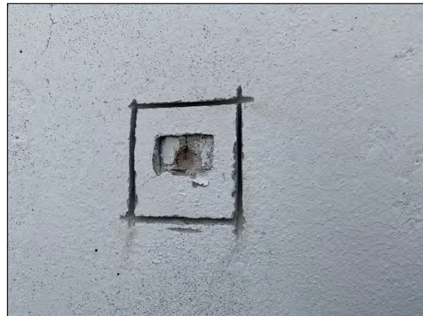
Concrete removal at south end of east parapet wall in progress.
