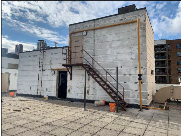
Concrete repair material applied on localized repair areas around mechanical penthouse.
