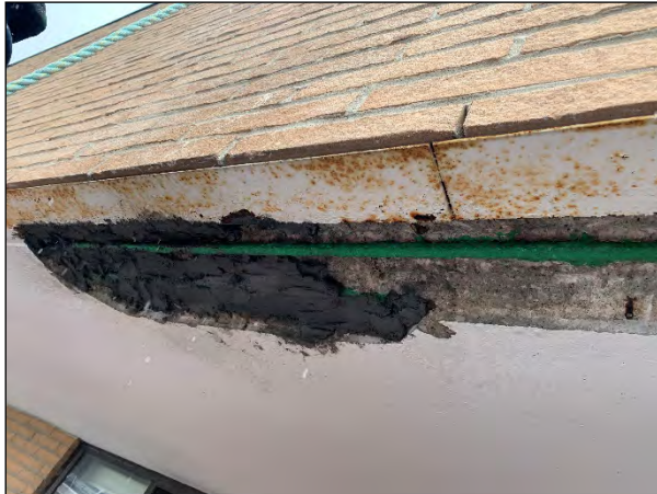
Installation of new sealants at window perimeters and soft joints along southern drop on east side of building.
