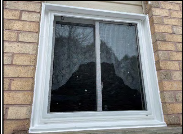
Exterior Finishing at New Windows
