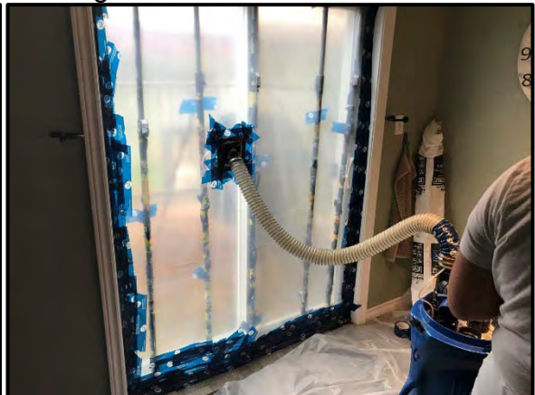
Testing of New Doors
