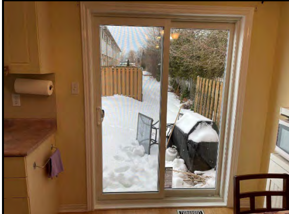
Interior Finishing at New Doors
