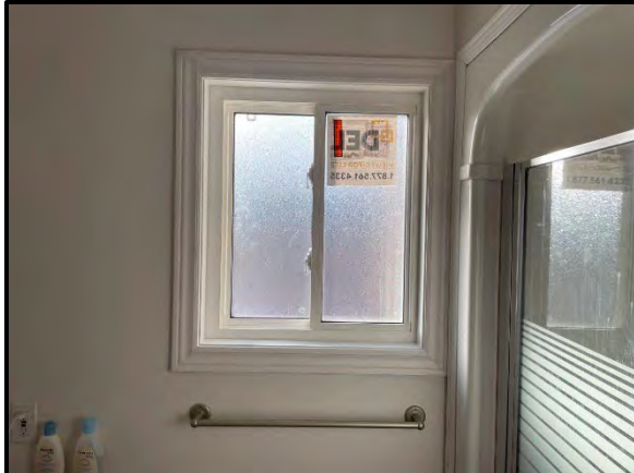
Interior Finishing at New Windows
