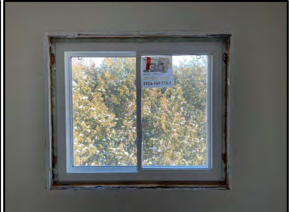
New Windows Installed
