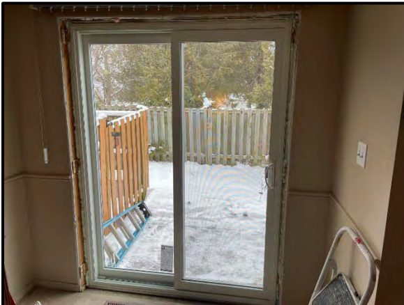
New Patio Doors Installed
