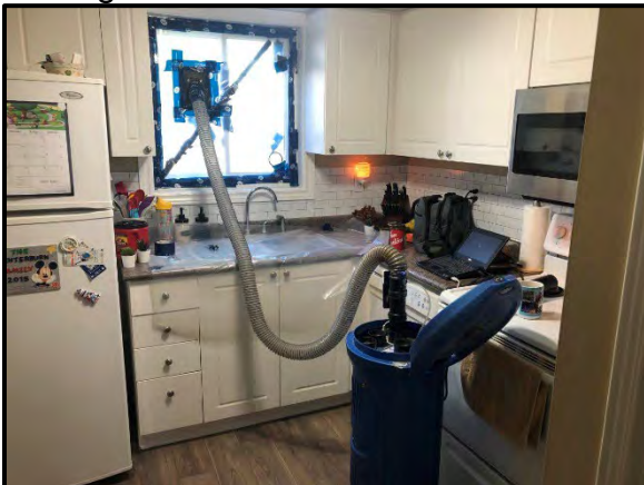
Testing of New Windows
