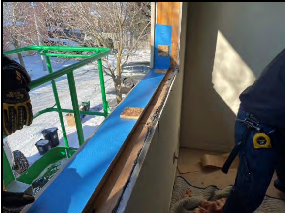
New Sub-Sill Flashing Membrane
