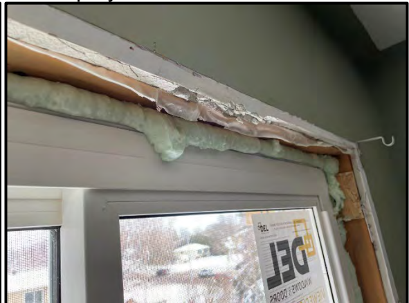
New Spray Foam Insulation within Cavities
