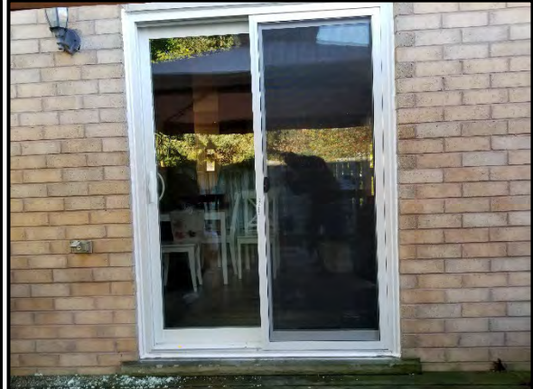
Exterior Finishing at New Doors
