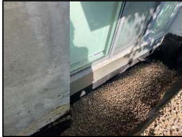
Backfilling in progress
