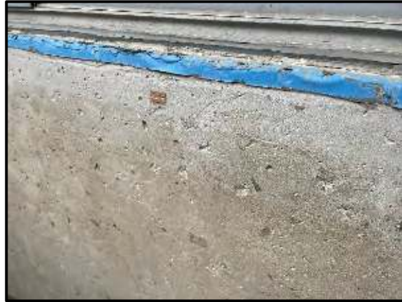
Surface preparation in progress
