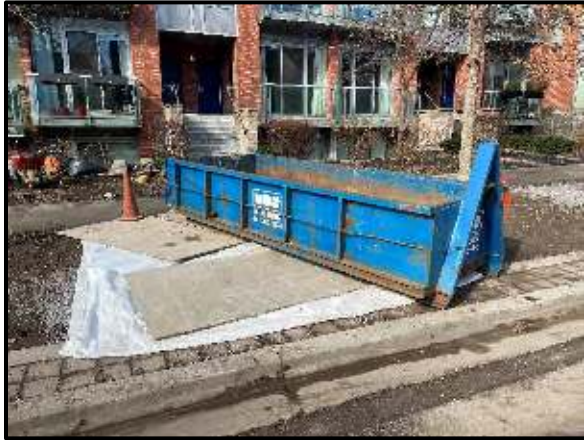
Removal of overburden material
