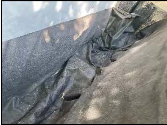
Filter cloth installation prior to backfilling
