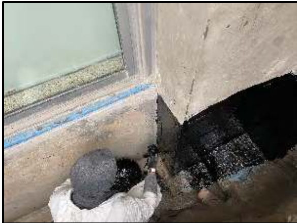
Installation of cold applied waterproofing
