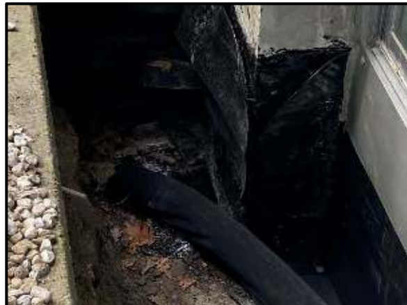
New weeping tile connected to old weeping tile
