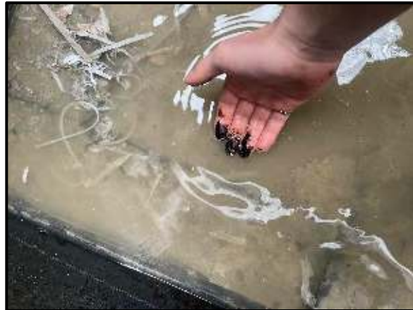
Water testing of the foundation
