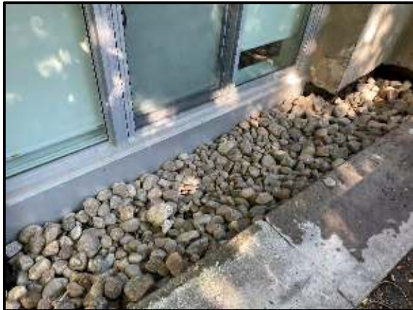
River rocks and backfill adjacent to the townhouse
