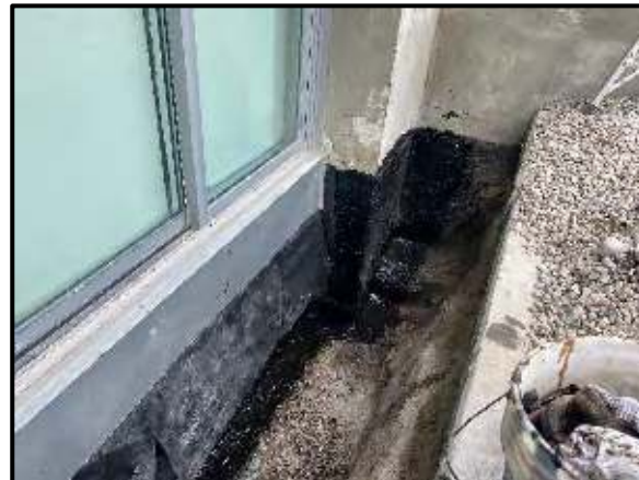
Cold applied waterproofing with aluminium flashings
