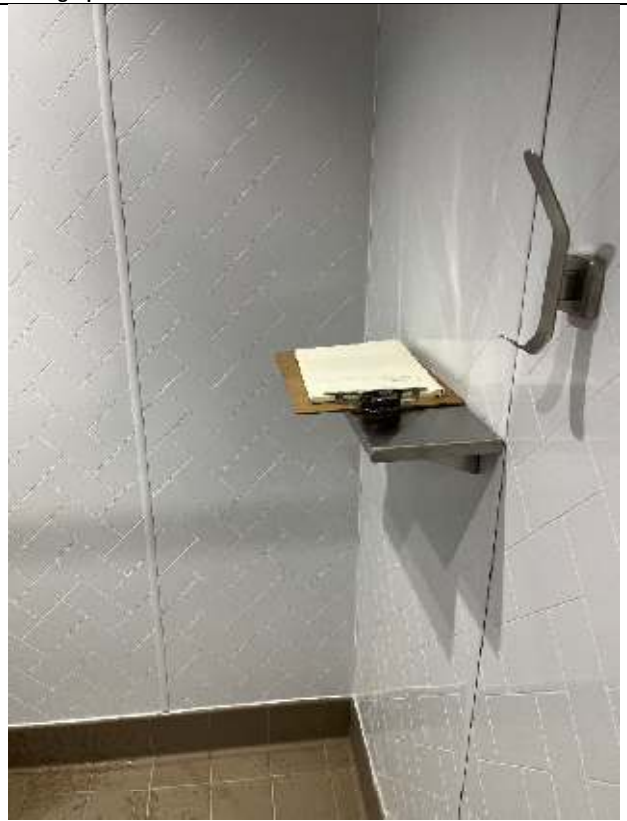
Photograph 8: Shelf and hook at New Shower 3
