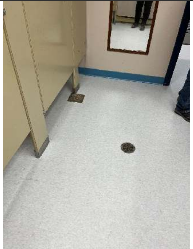
Photograph 4: New flooring and base at Washroom 1
