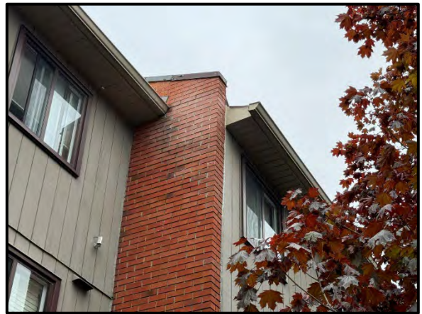
Localized Replacement of Deteriorated Bricks at the Chimney Walls.
