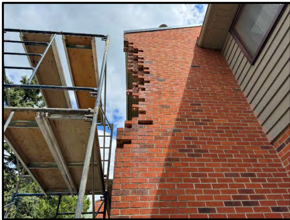
Localized Removal of Deteriorated Bricks at the Chimney Walls.
