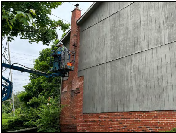
Localized Removal of Deteriorated Bricks at the Chimney Walls.
