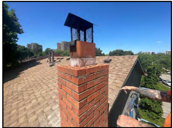
Localized Replacement of Deteriorated Bricks at the Chimney Walls.
